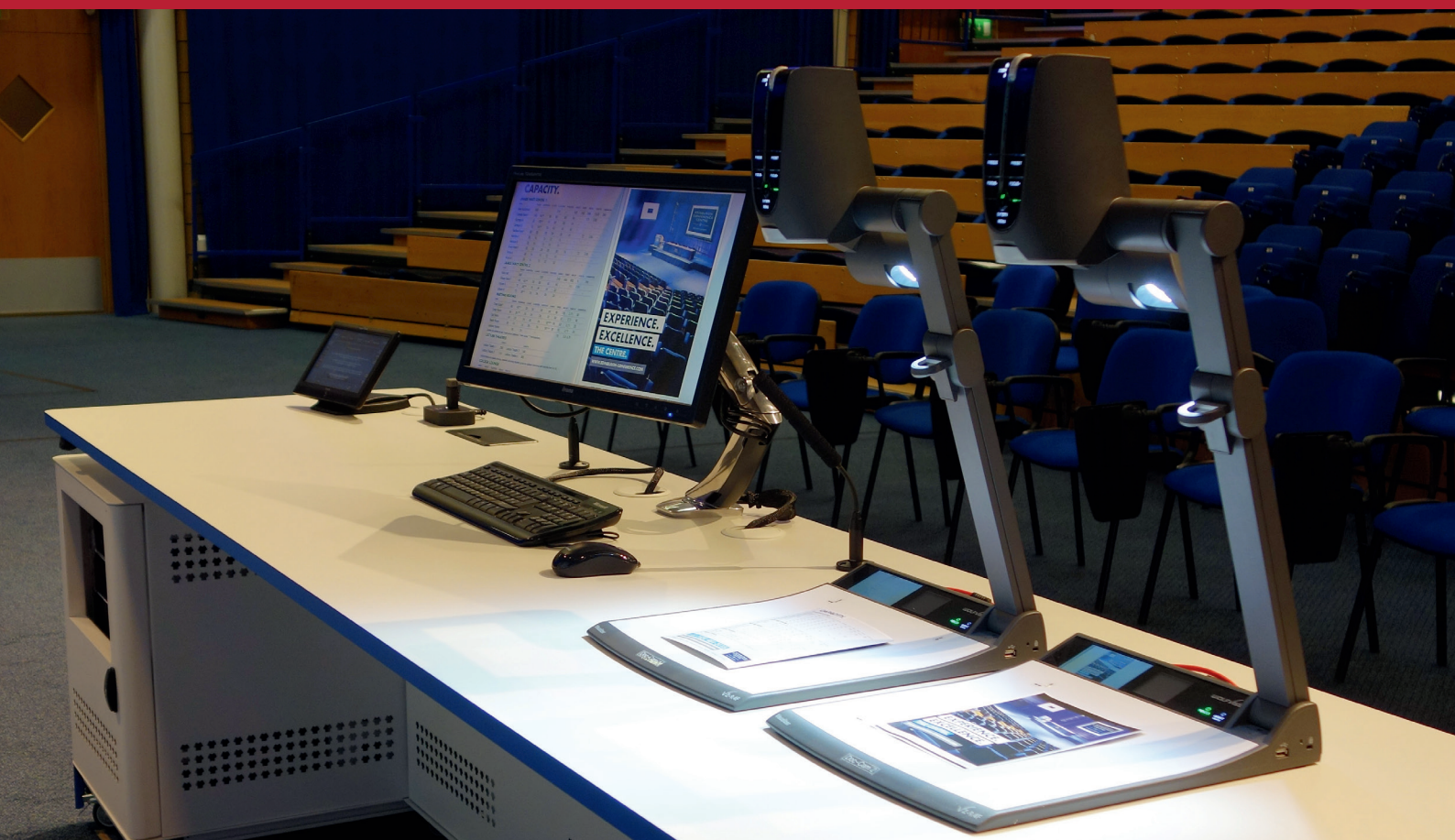
Two WolfVision VZ-9.4F Visualizers installed side by side at Heriot-Watt University.
