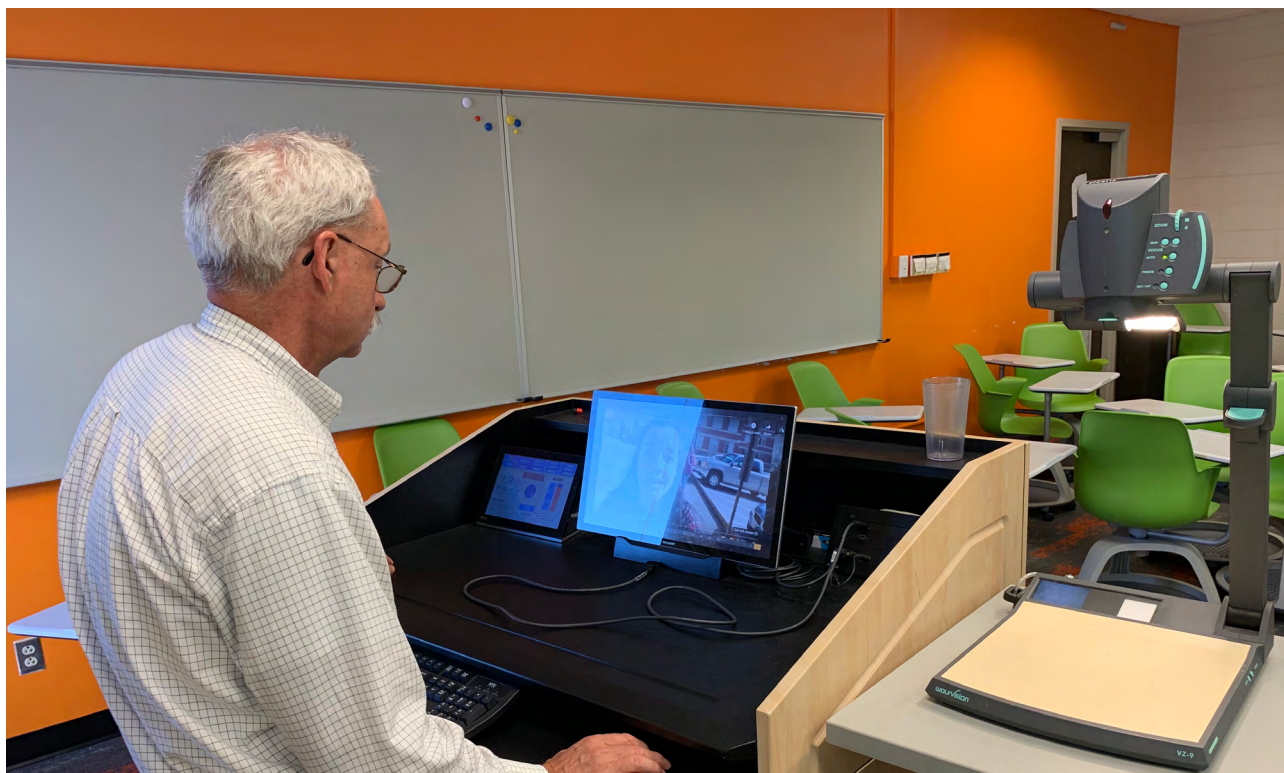
View from the lectern equipped with Cynap, touchscreen controller, AMX control panel and WolfVision Visualizer.
