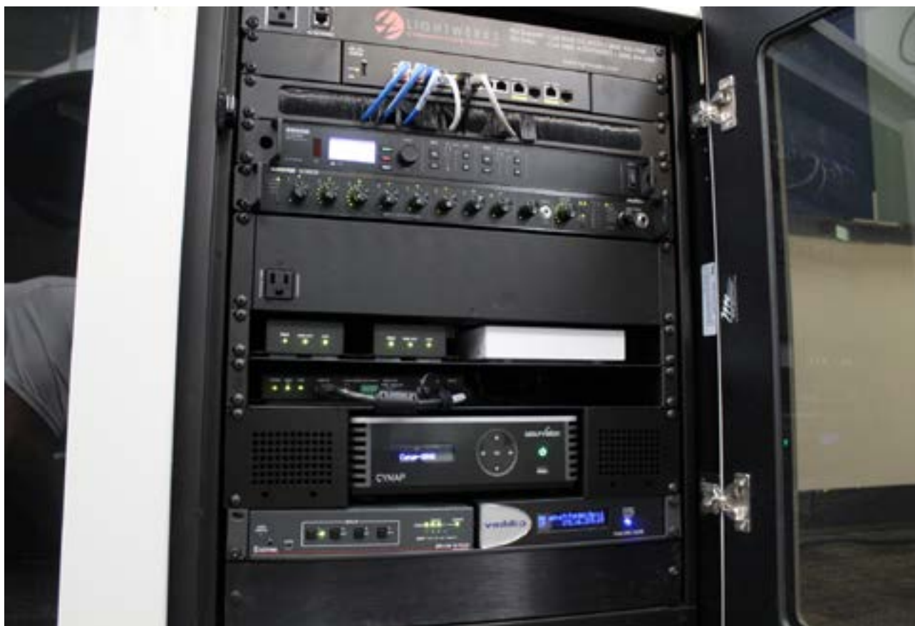
Rack-mount installation of WolfVision Cynap at SRHD.
